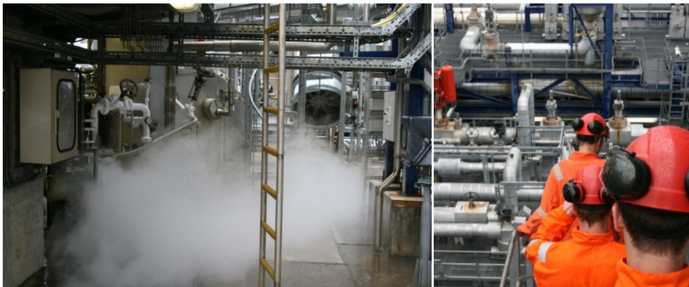
Figure 2. A typical oil and gas plant environment.
